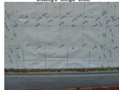
STEP #5 Tape existing and new Tyvek on all four sides.
