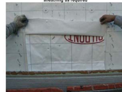
STEP #4 Attach the new slip sheet onto sheathing
