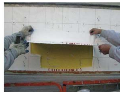
STEP #3 Slip new sheet of Tyvek under existing Tyvek – extend 6" up Creating a "shingle" effect
