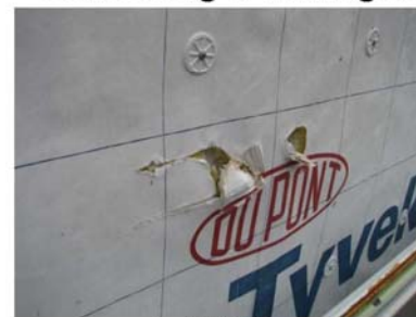
STEP #1 Hole or tear is identified
