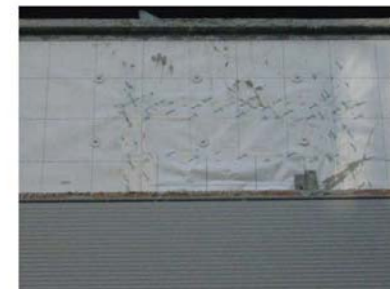
STEP #6 Install gasketed screws a minimum 16" o.c. – both directions (into studs)
