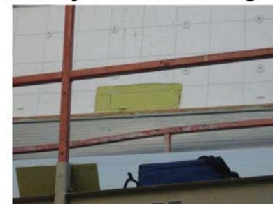
STEP #2 Cut & peel up Tyvek (4" above tear) and replace damaged sheathing as required
