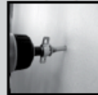
3. Use a standard drill drive for 5/16 hex head
