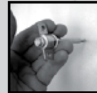
1. Line Up screw at stud location
