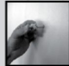
2. Push screw into insulation as far as possible with your hand
