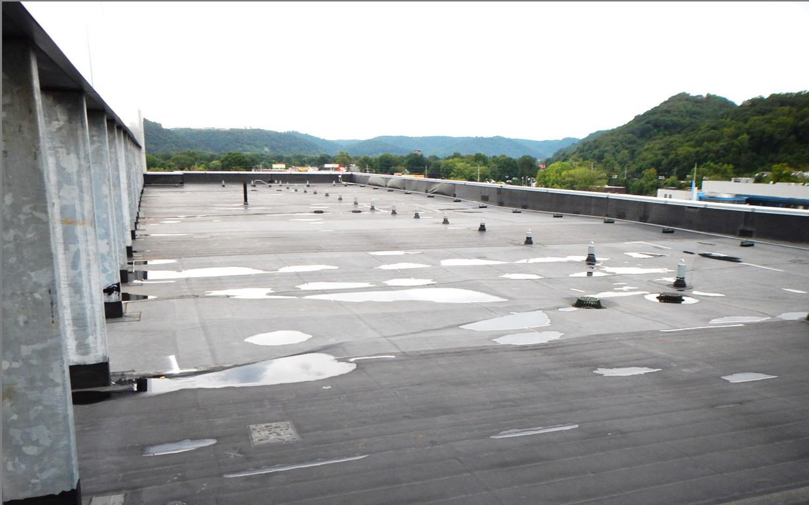
View of roof area following a storm event, where ponding areas and insulation deformation is more evident.
