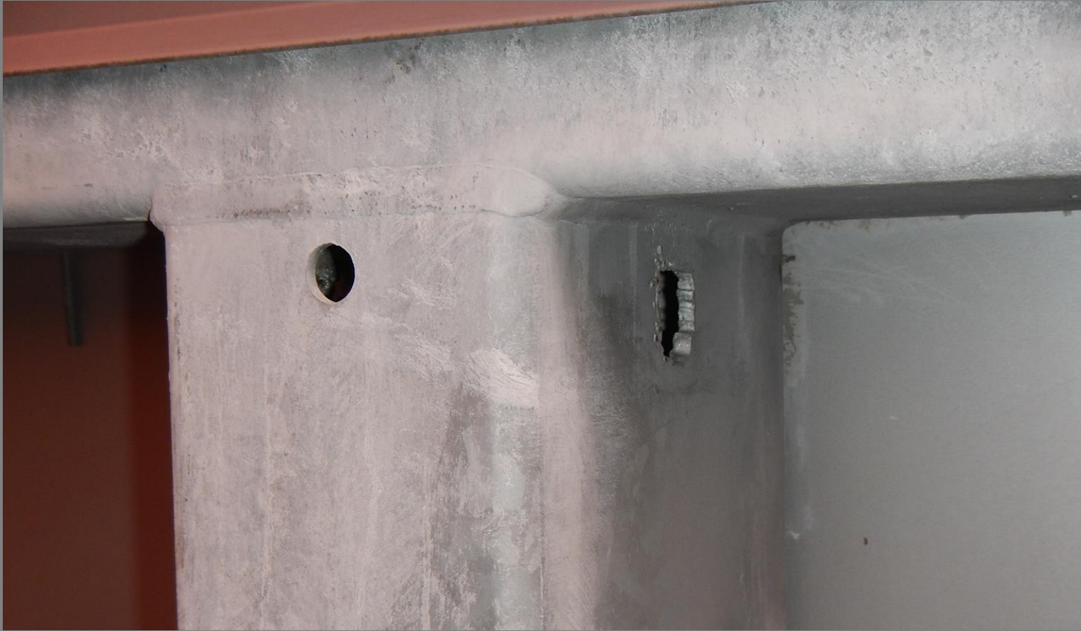
Close-up view of exposed drain holes in the galvanized steel columns allowing direct water infiltration and air exfiltration. Note some holes are drilled and some are cut with a torch.
