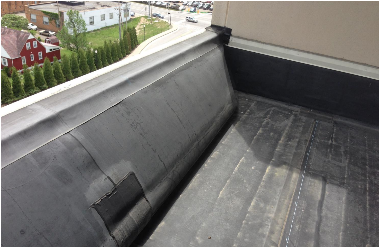
View of parapet wall where membrane is ballooning out and has deboned from the pre-cast concrete wall.
