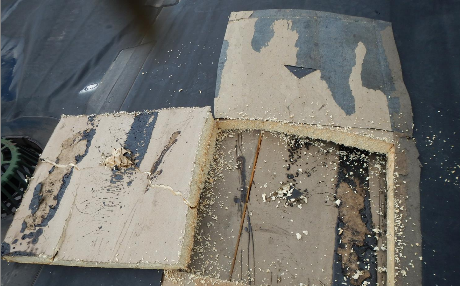
View of poor interlayer adhesion between insulation boards.
