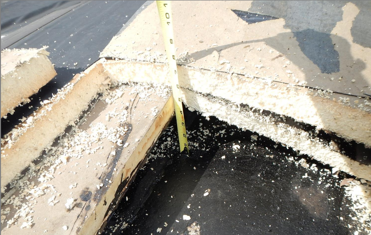
View of deformed polyisocyanurate insulation.
