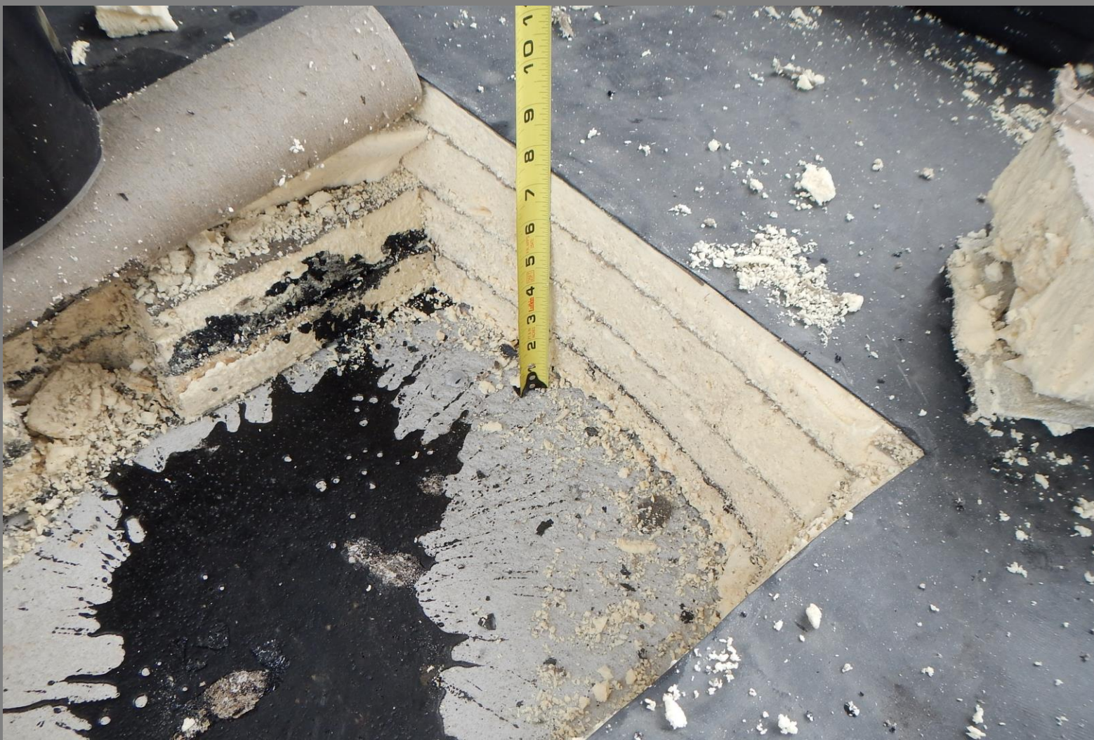
View of poor asphalt coverage on concrete deck
