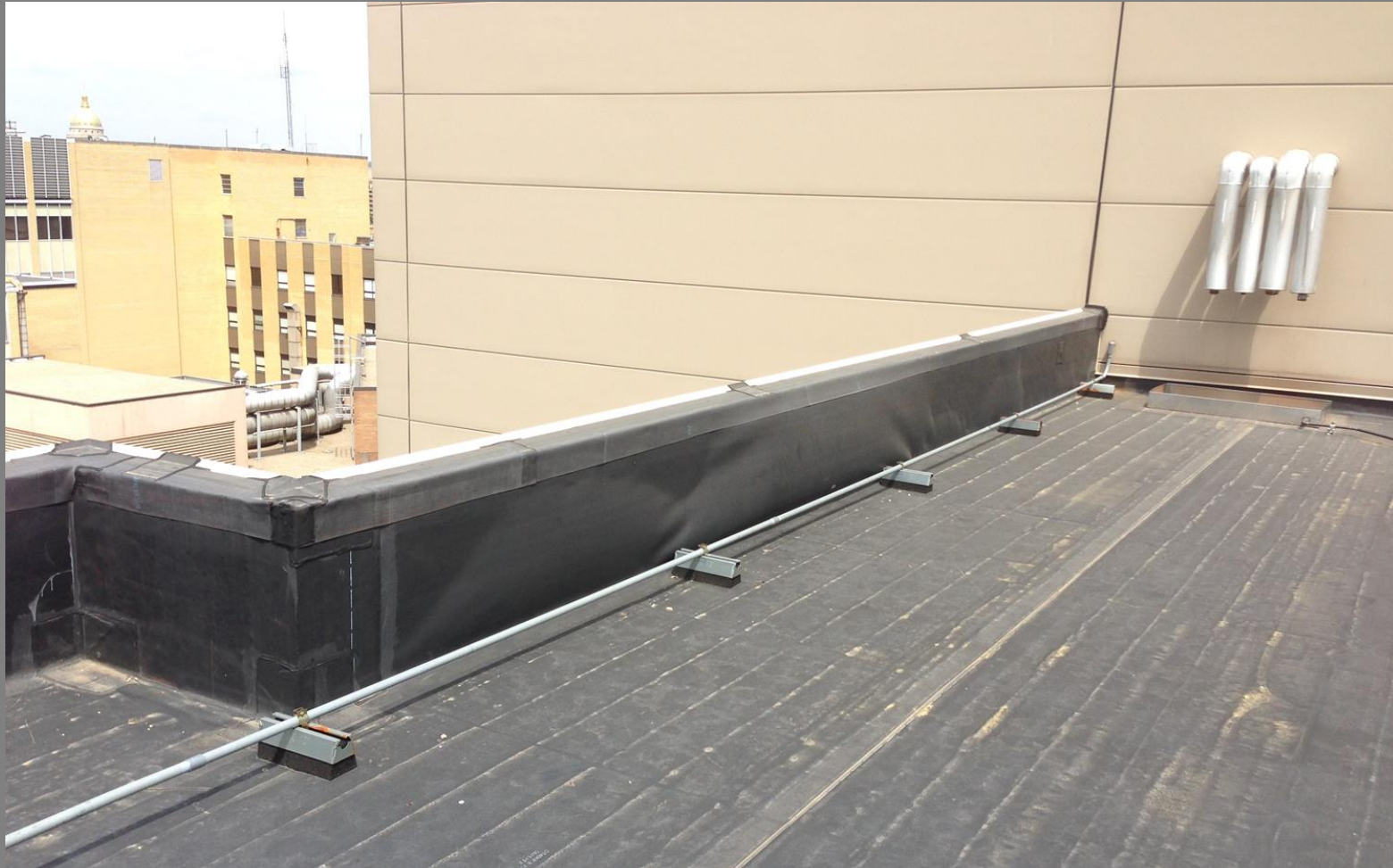
View of a parapet wall where EPDM membrane has debonded from the wall surface.
