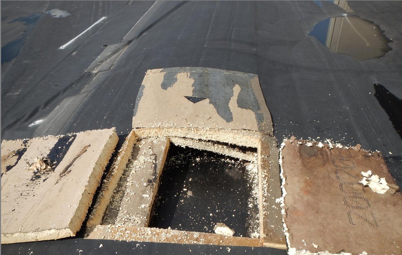
View of large deformation in the insulation, note evidence of water staining even though insulation was dry.
