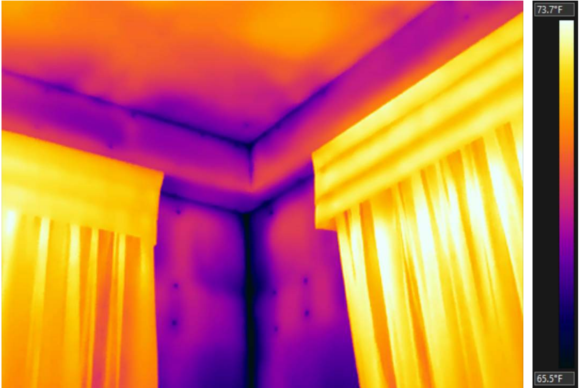
Cool Spots due to poor air circulation
