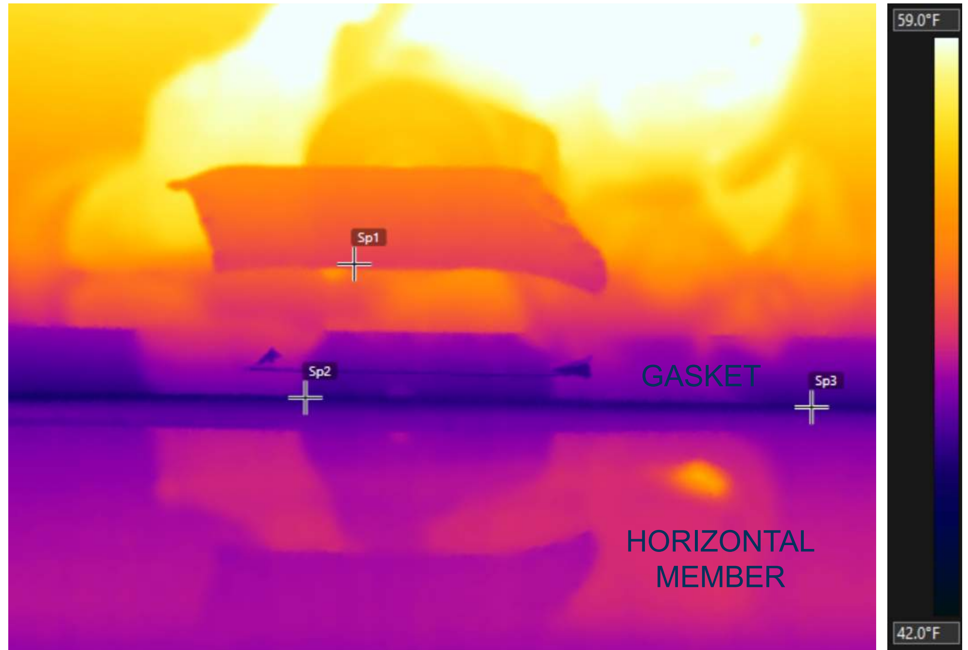
NICU Room 14 – Interior at Middle Tube
