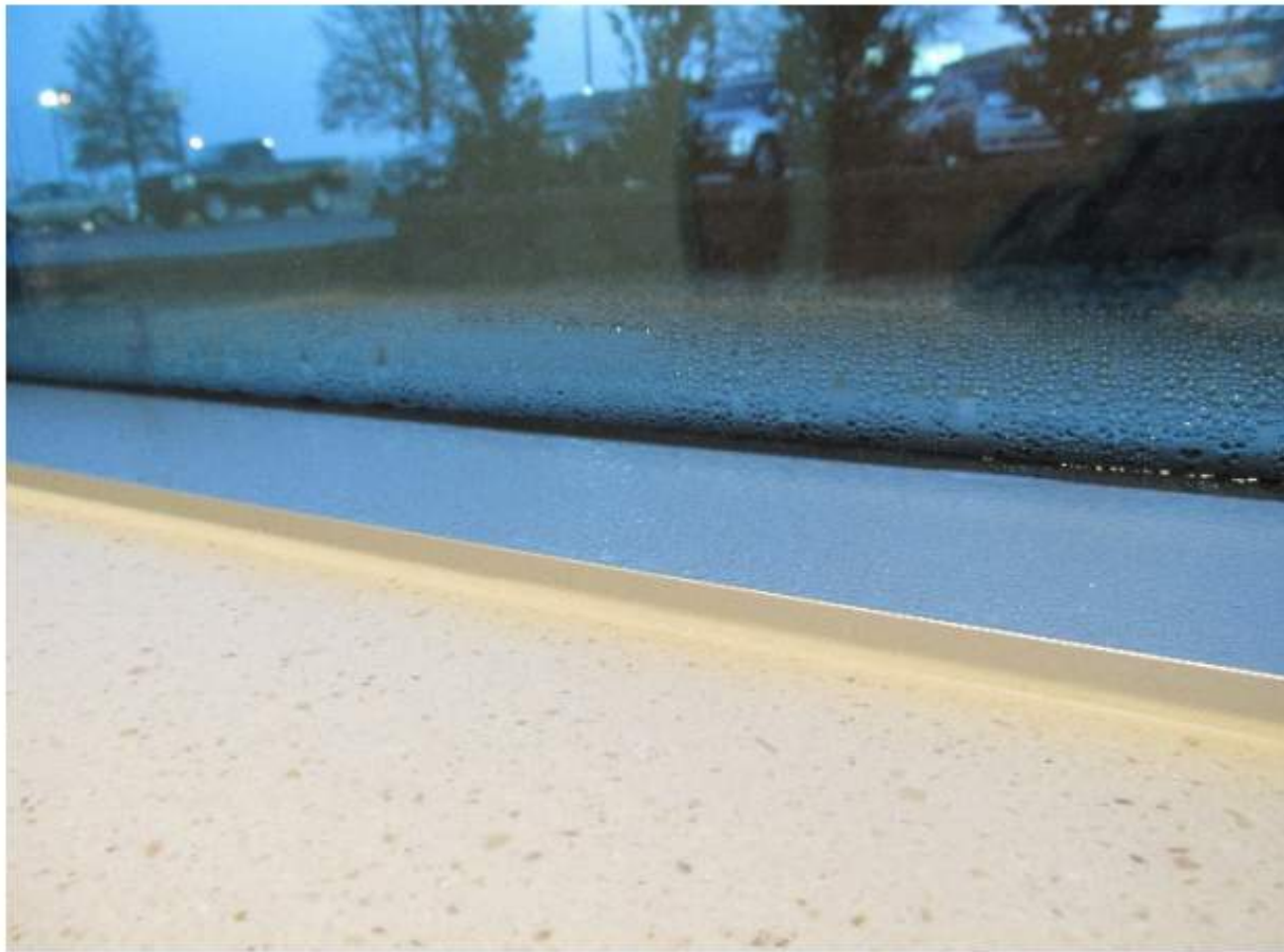
NICU Room #14: Image on left was taken upon arrival at 7:15am on 2/2/18. Image on the right was taken to document the reoccurrence of condensation within 30 minutes of drying glass and tube.
