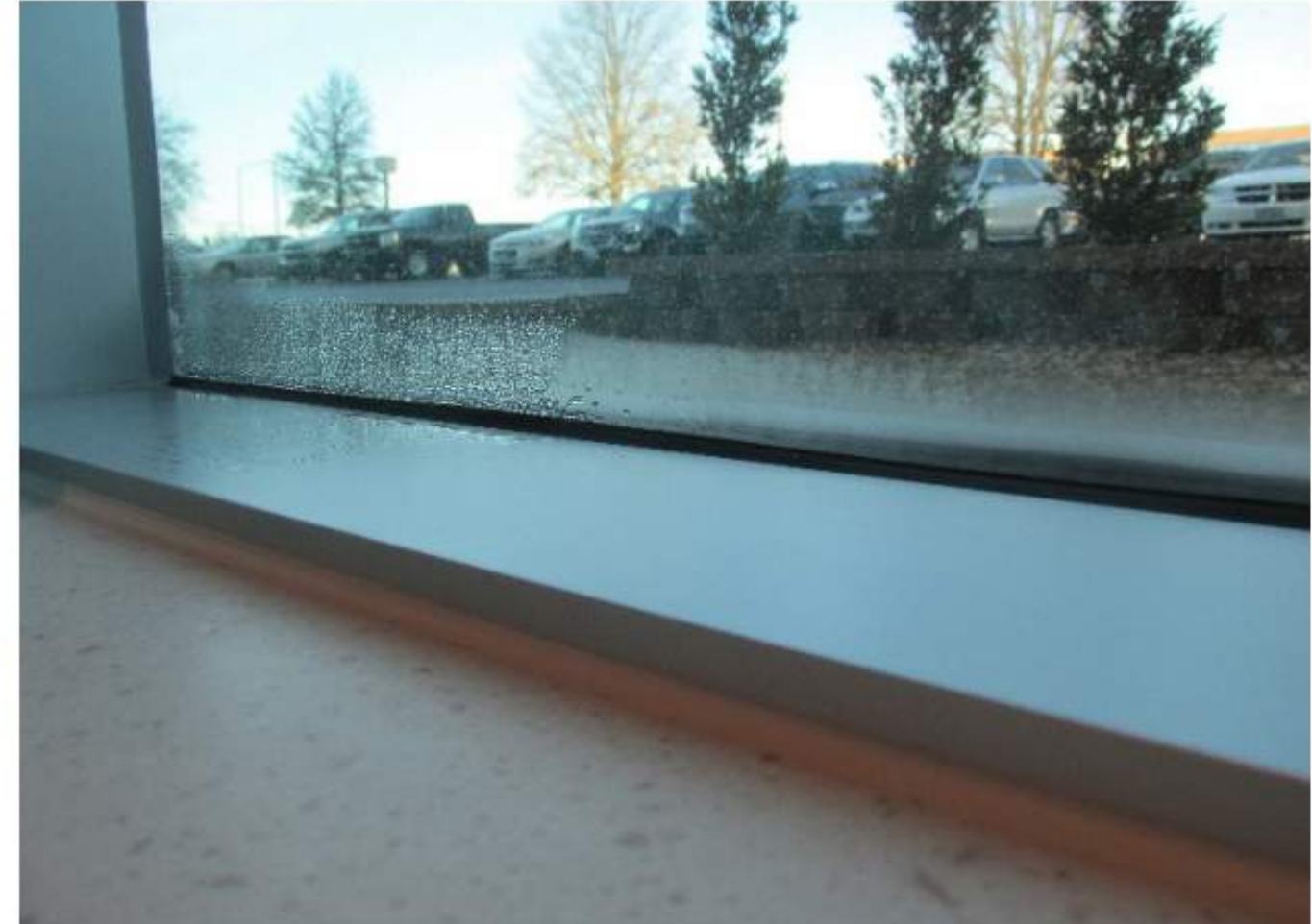
NICU Room #14: Image on left was taken upon arrival at 7:15am on 2/2/18. Image on the right was taken to document the reoccurrence of condensation within 30 minutes of drying glass and tube.
