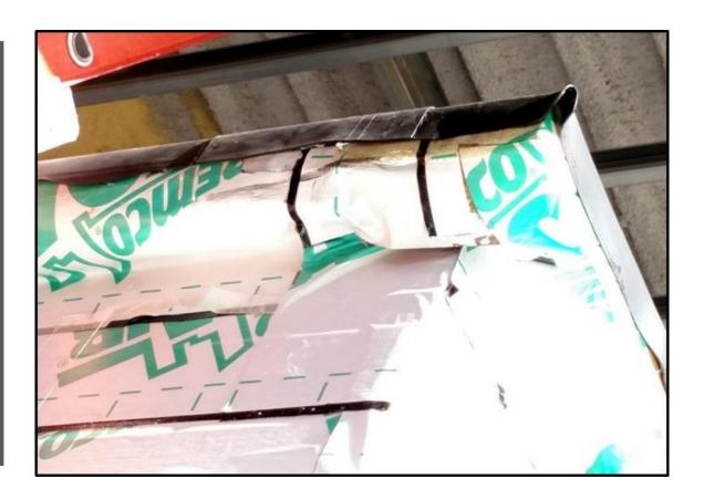
Most common location of air and water leakage is the parapet
