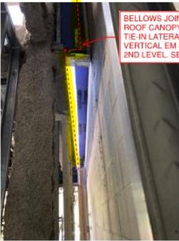
Location 2: Expansion joint at canopy
