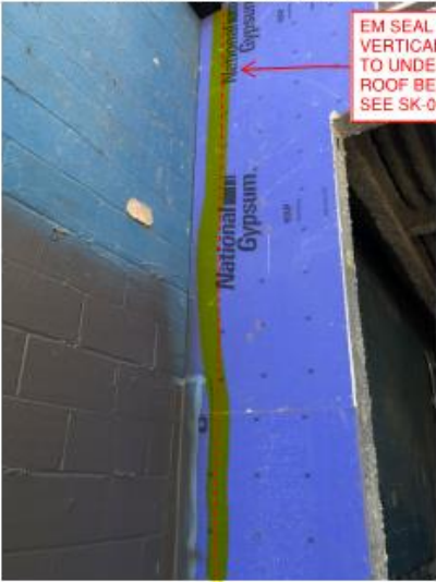
Location 3: Vertical expansion joint
