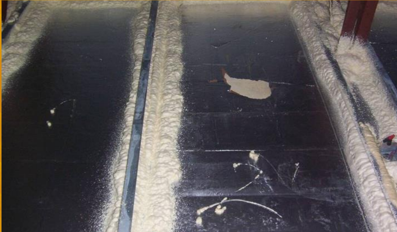
Metal soffit panel seams, sealed with foam sealant
