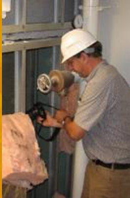
Trained Assessor with camera, floor plans and intake form or Air Leakage Data Collection APP
