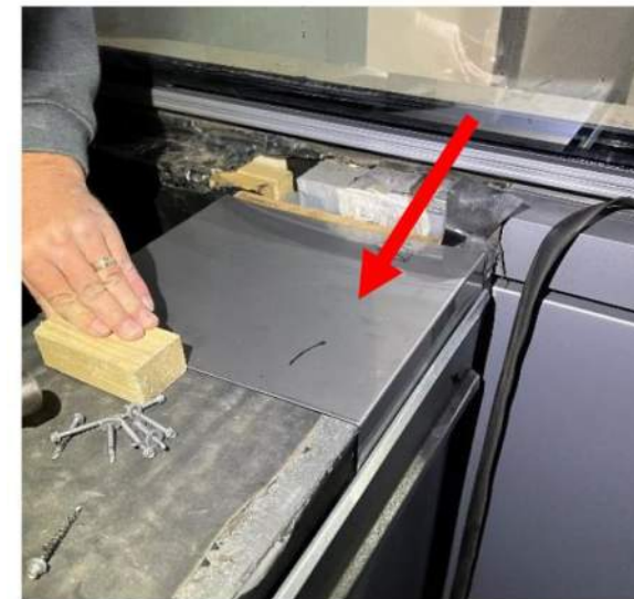
Figure 9.1c – Stainless steel saddle flashing installed at parapet.
