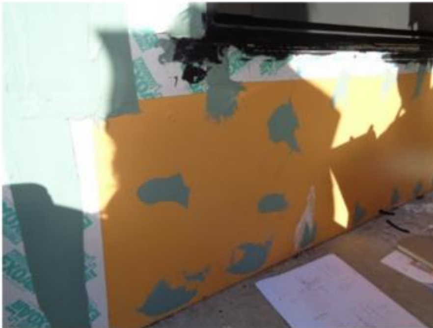
SV.01.02.A - Fasteners covered with Dymonic 100.
