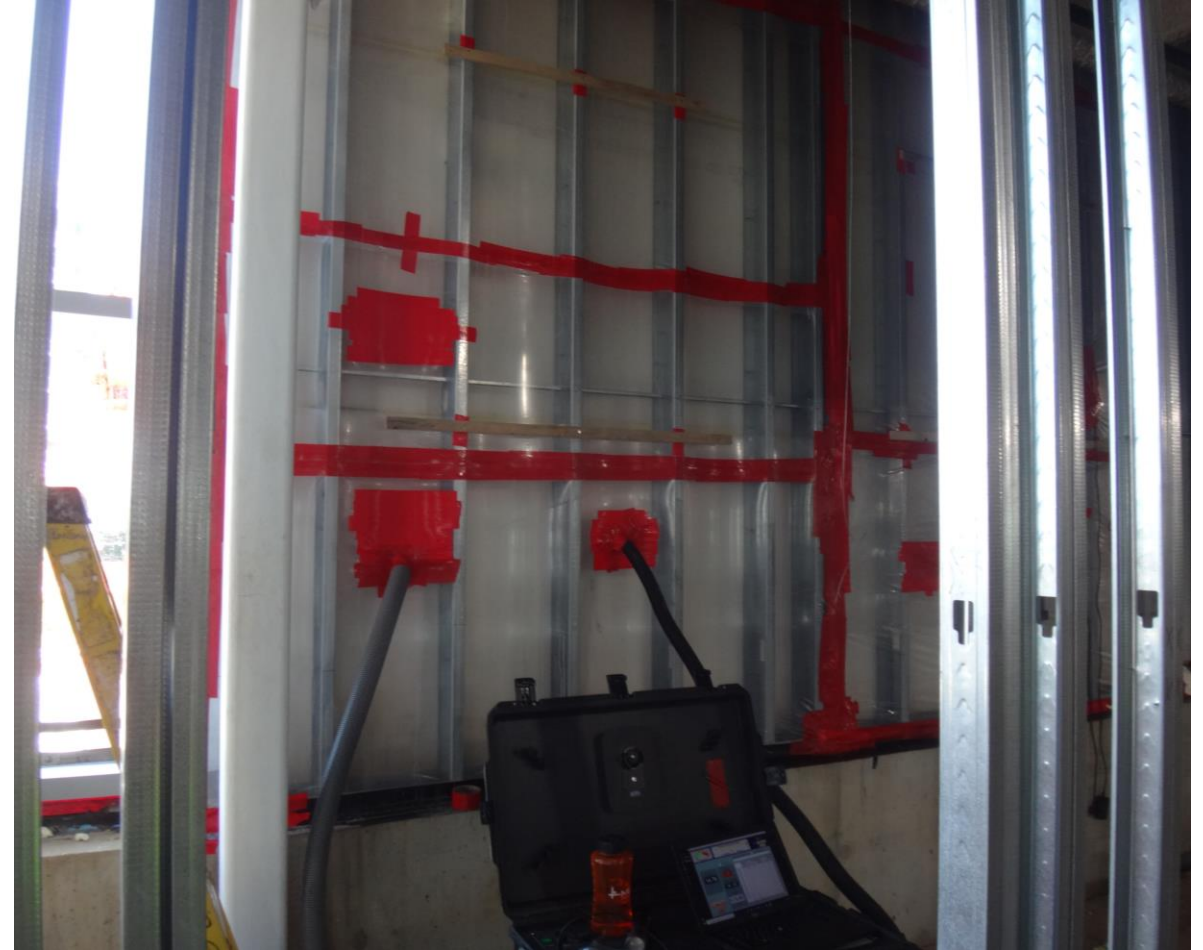
Interior View: Pressure Chamber
