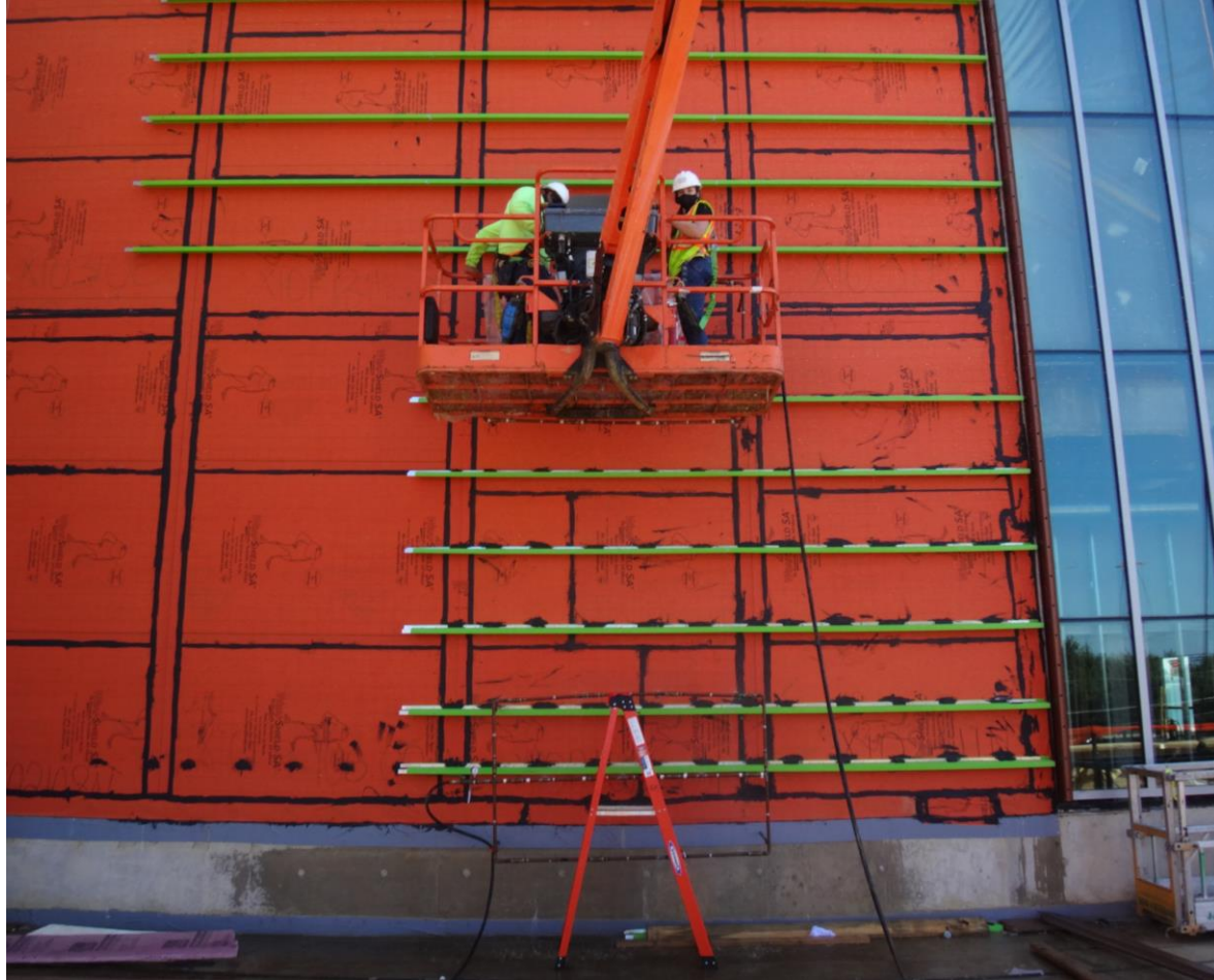
Exterior View: Water Testing
