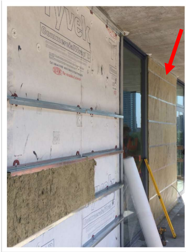
Exterior Insulation Attachment Mockup
