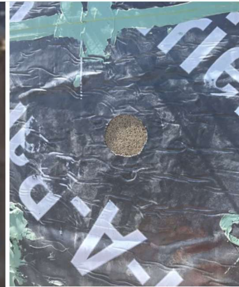
View of test location #1
