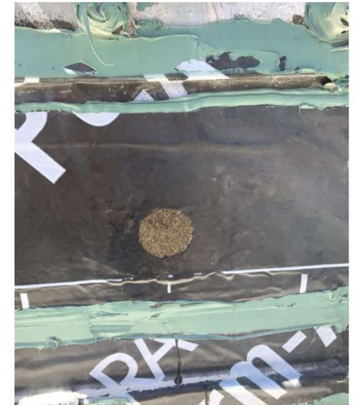
View of test location #2
