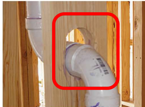
FIGURE 19: Example detail and photo showing the hole in a wood stud added to accommodate shrinkage around plumbing
