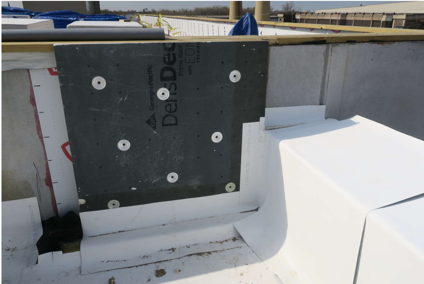
Roof (Horizontal) Condition
