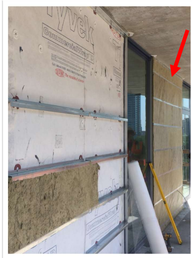
Exterior Insulation Attachment Mockup
