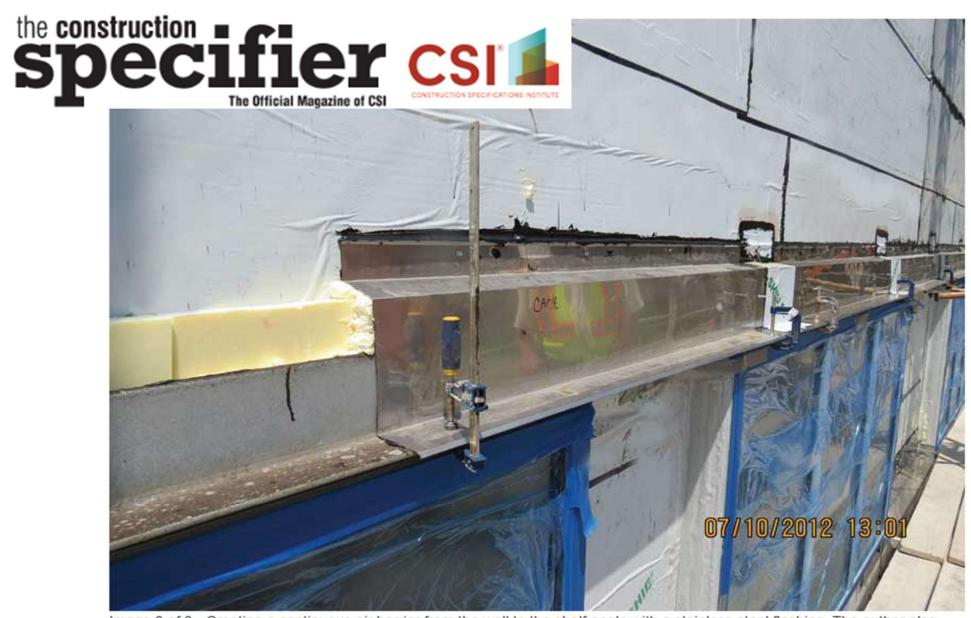
Image 3 of 3 - Creating a continuous air barrier from the wall to the shelf angle with a stainless steel flashing. The author also installed a spray polyurethane foam (SPF) solid under the stainless steel flashing to reduce the condensation potential under the flashing.
