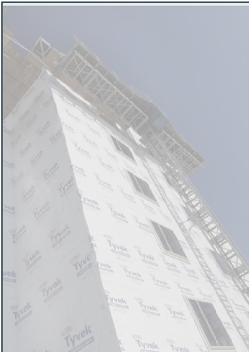
Mechanically Fastened Air and Water Barrier Systems offer outstanding protection for gypsum, CMU, and many common sheathing substrat
