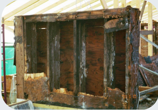
FAILURE AT ROOF PARAPET
