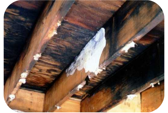
FAILURE AT SOFFITS AND DECKS
