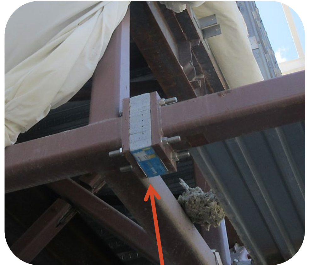
Thermal isolator pad at steel canopy support
