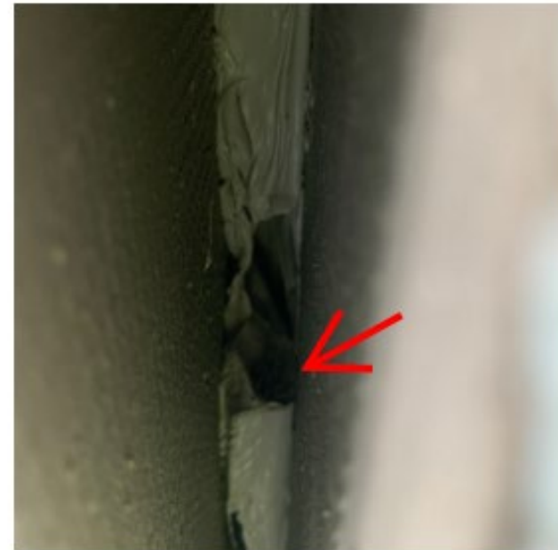
Unsealed Splice Between Panels 10-17 and 10-18
