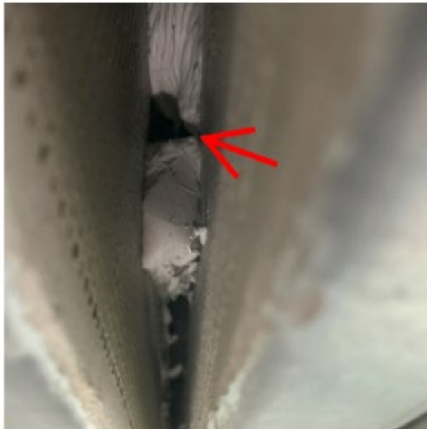
Unsealed Splice Between Panels 10-11 and 10-12
